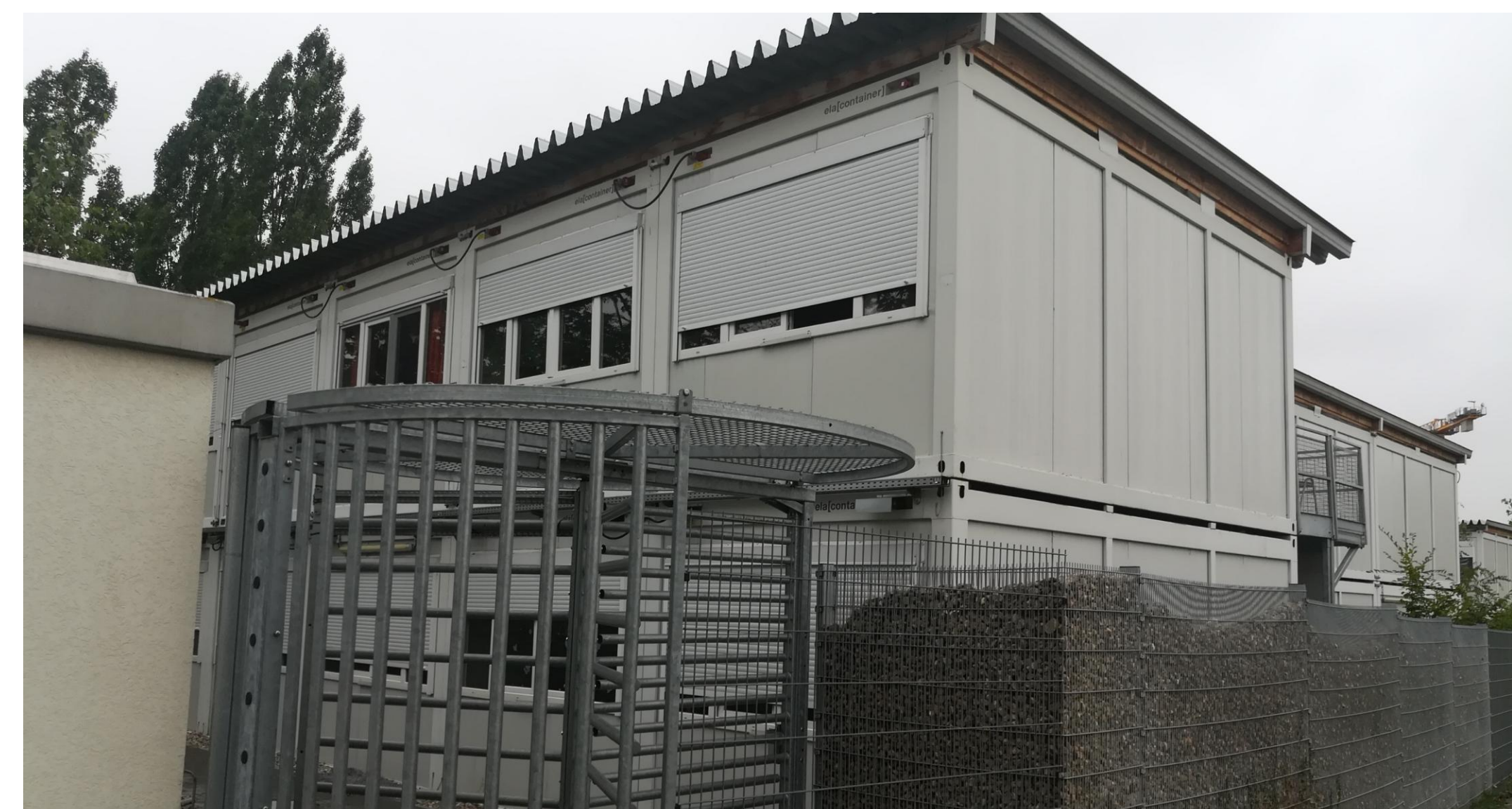
Fig. 1 A satellite facility of a large asylum reception centre in Ingolstadt, Germany, built from modular containers (Photo: Anna Huber)
